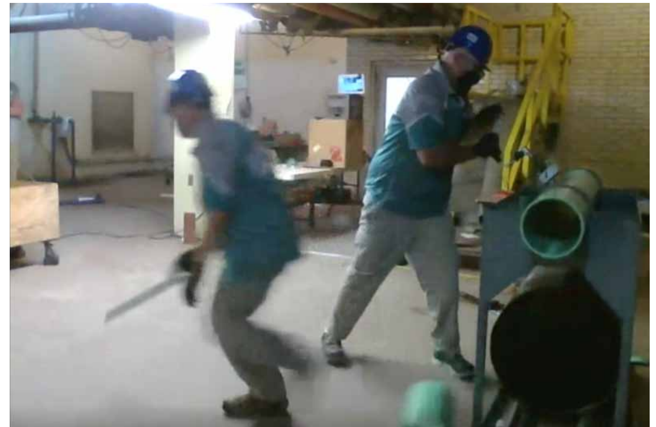
Lofaro scrambles to retrieve a tool while Burnette vigorously cuts into a pipe during the Collections Systems Event. Image courtesy of WEF
