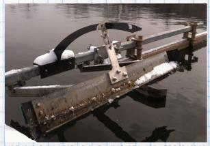
LIFTING THE SKIMMER ARM UP USING THIS HOOK PREVENTS IT FROM FREEZING TO THE TROUGH. THIS INGENIOUS FIX MAKES THE MOST OF EASILY AVAILABLE AND SAFE TOOLS AND IS QUICK, SAFE, AND SIMPLE TO USE. James Spielvogel
